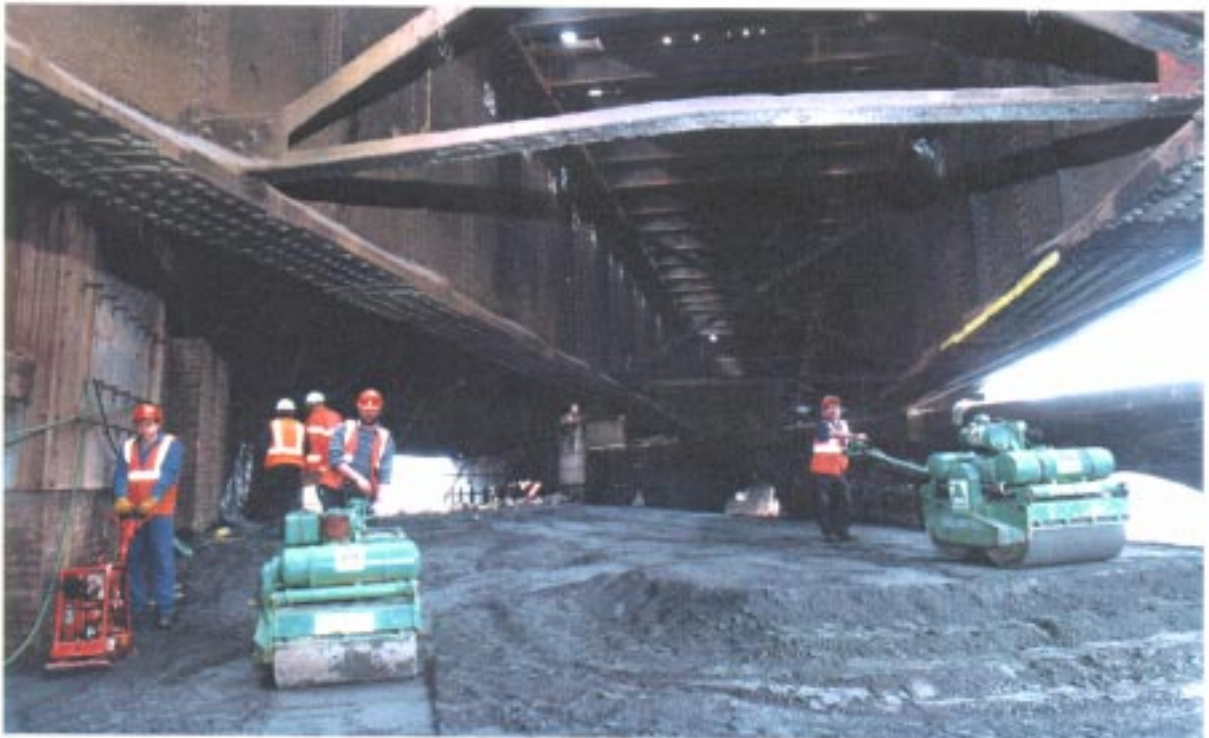
COMPACTION OF PFA BENEATH BRIDGE STRUCTURE
