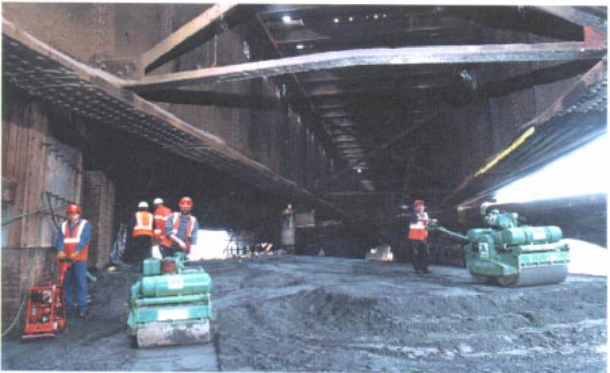
COMPACTION OF PFA BENEATH BRIDGE STRUCTURE
