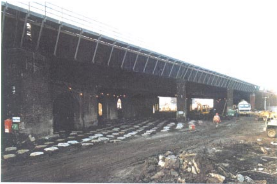
PILES INSTALLED BENEATH THE BRIDGE STRUCTURE
