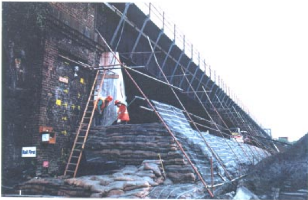
VIEW OF EAST SIDE EMBANKMENT UNDER CONSTRUCTION
