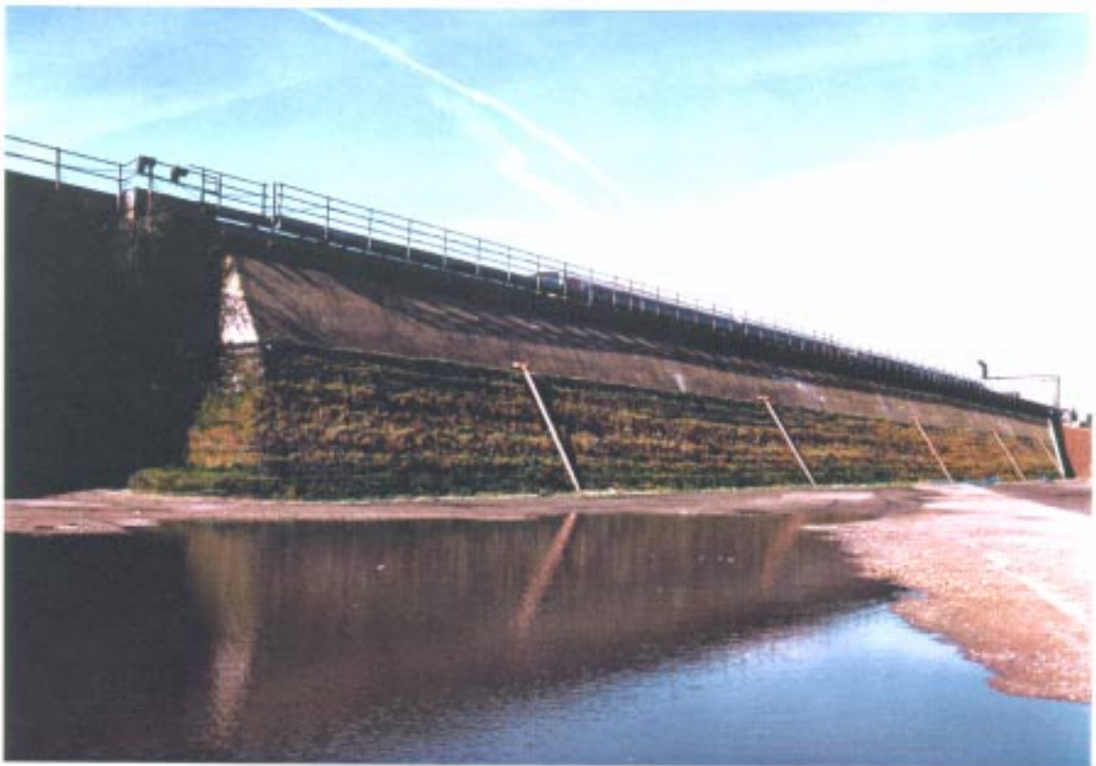
VIEW OF COMPLETED EMBANKMENT
