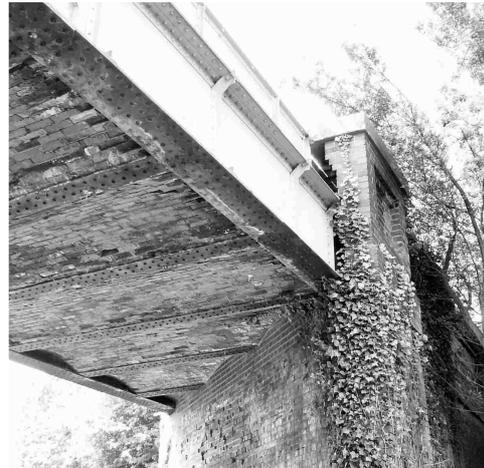
Figure 5 Typical Half Through Girder Bridge on Masonry Abutments
